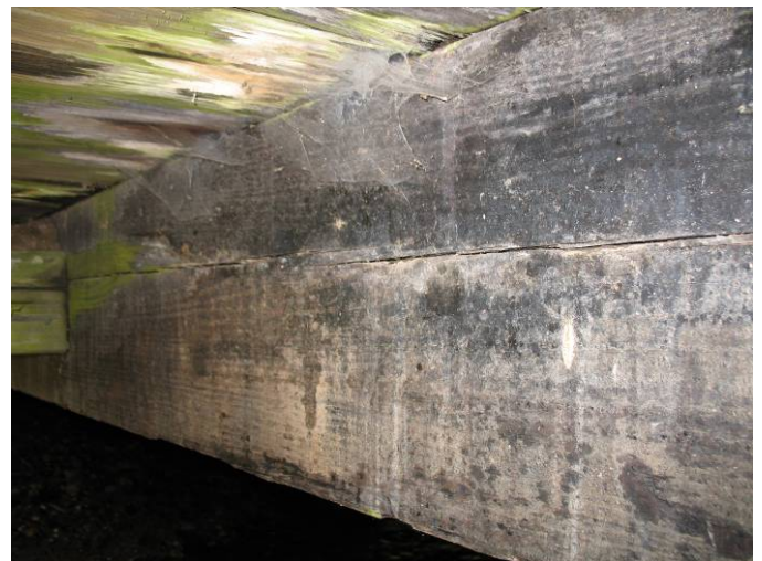
Figure 200. Checking in the Girders
