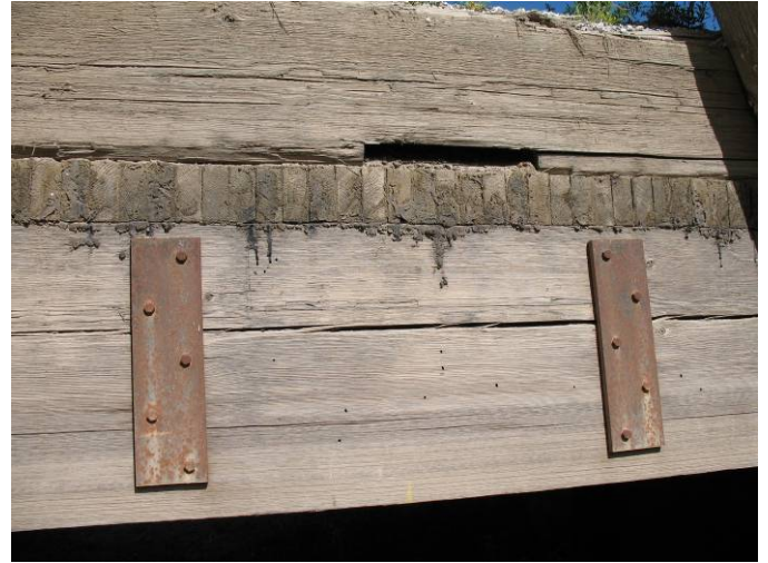
Figure 350. Checking in Exterior Girders
