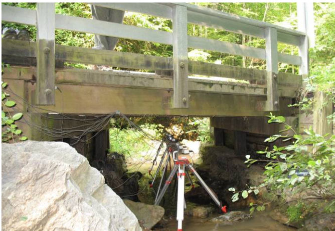
Figure 32. Madison County Parapet
