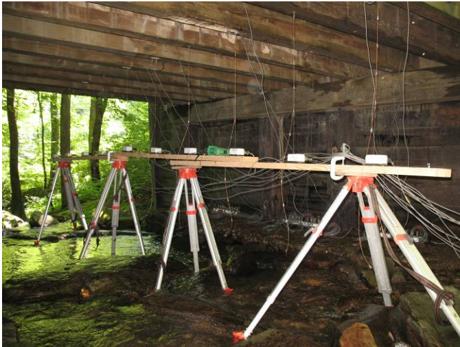
Figure 100. Typical Deflection Instrumentation
