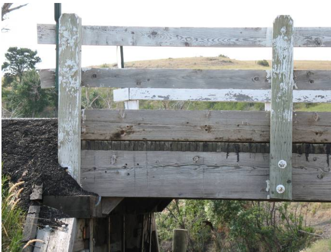
Figure 367. Montana Bridge Parapet Support
