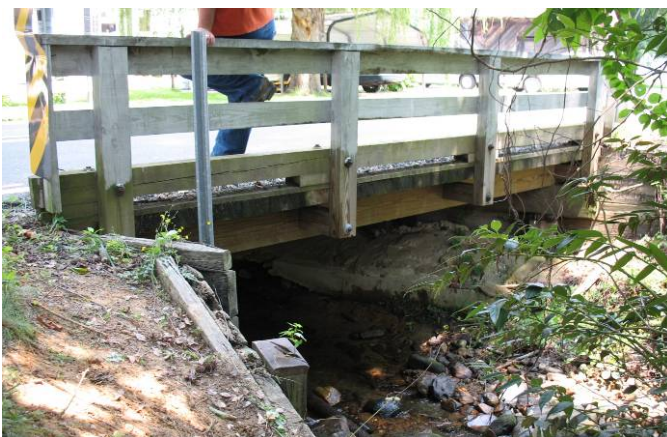
Figure 218. McDowell County Parapet Support
