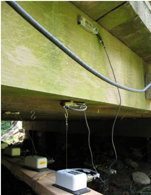
Figure 161. Outside Girder Strain Transducer Setup
