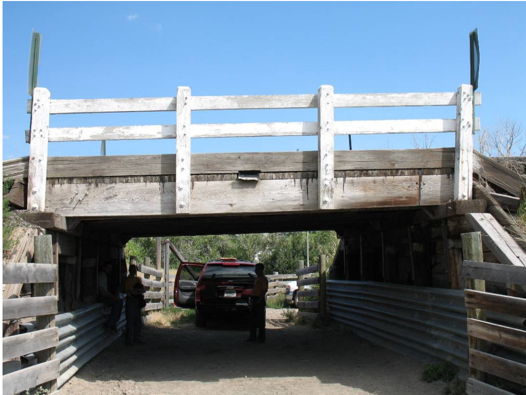
Figure 13. Montana Bridge used for Finite Element Modeling
