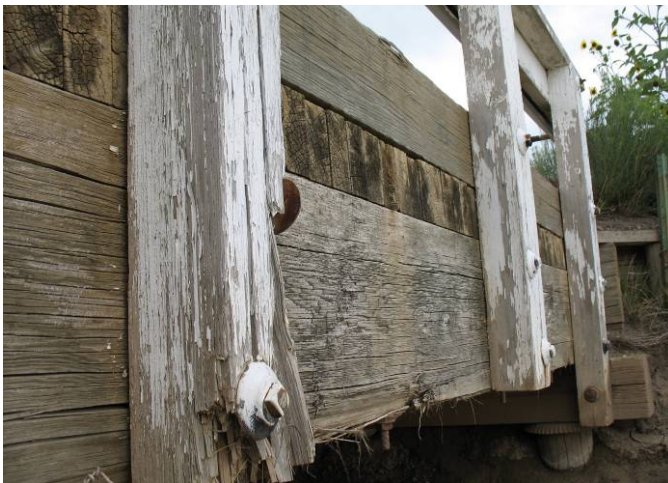
Figure 276. Colorado Bridge Parapet Support
