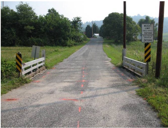
Figure 61. Red Horse Creek Bridge
