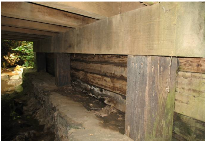
Figure 31. Substructure Sill and Columns
