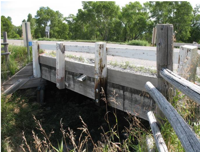
Figure 338. Montana Bridge Parapet Support
