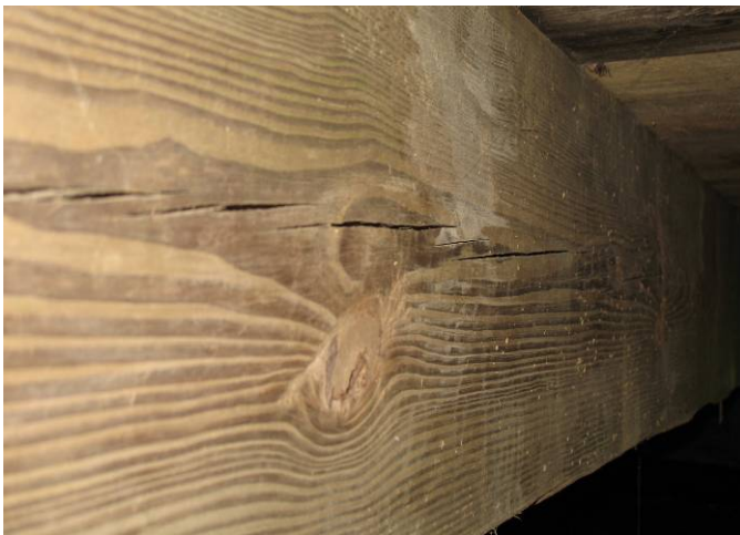
Figure 44. Checking at Centerline of Girder
