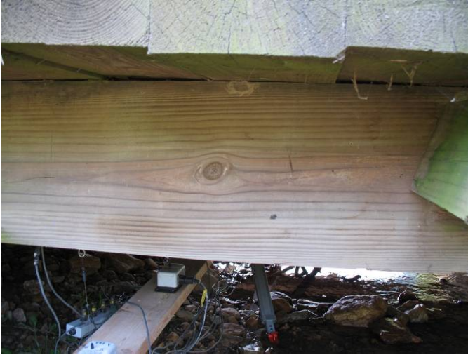
Figure 73. Deck Board Detachment
