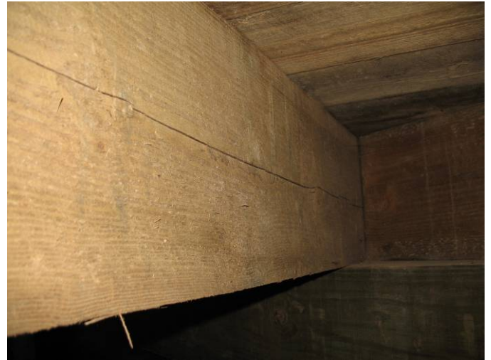
Figure 45. Checking at Centerline Near Abutment
