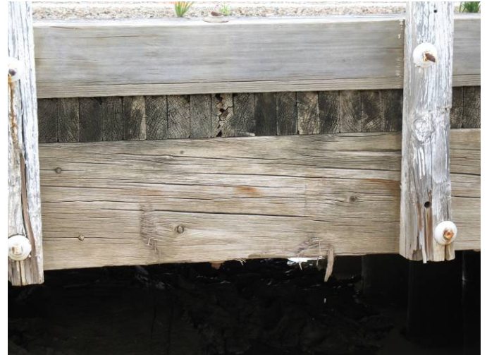
Figure 287. Checking in Exterior Girders
