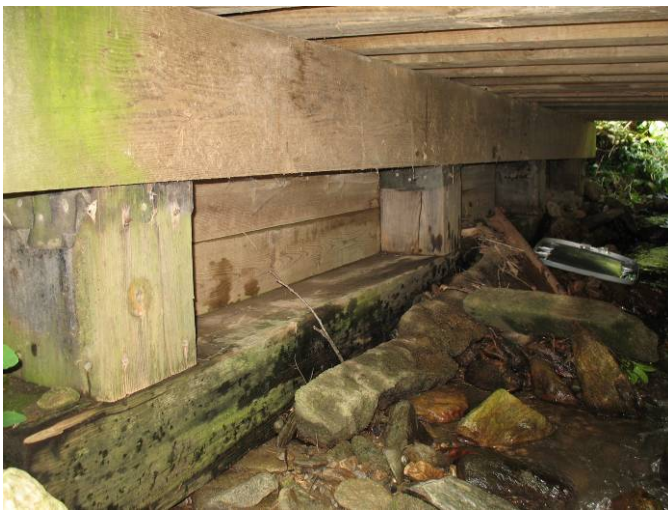
Figure 97. Madison County Bridge Substructure
