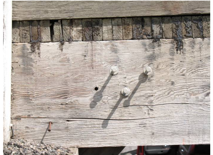
Figure 378. Checking in Exterior Girders
