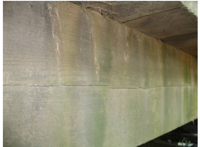
Figure 139. Checking at Girder Centerline
