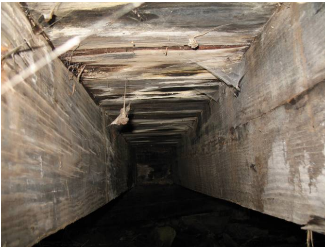
Figure 197. Girder and Deck Condition
