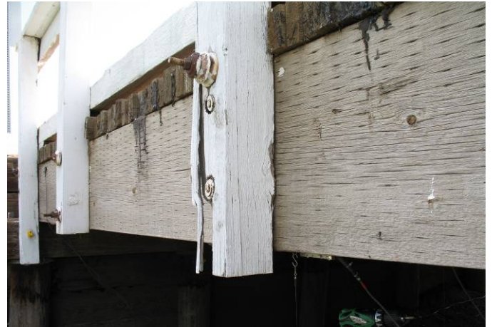
Figure 259. Exterior Girder Condition
