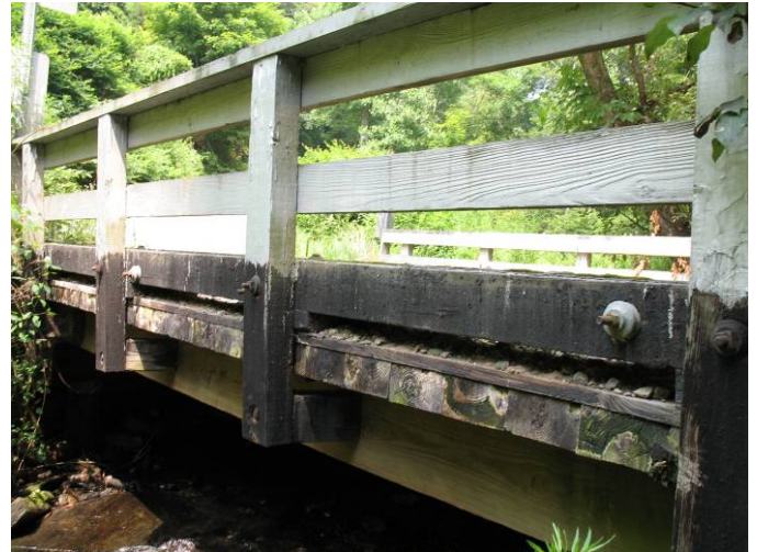
Figure 186. Doebag Creek Parapet
