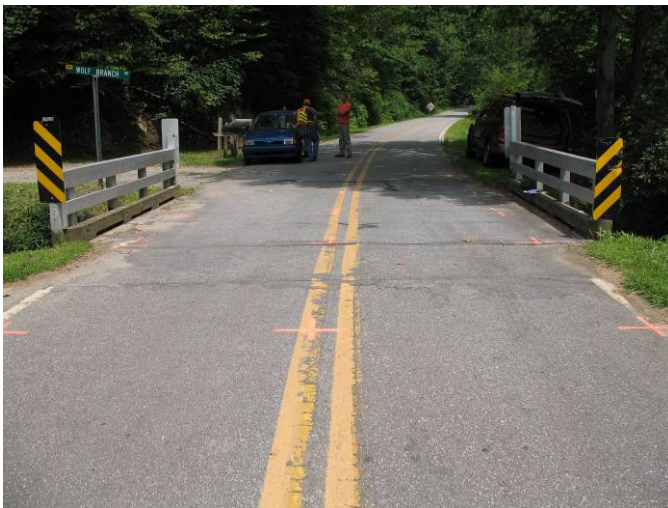
Figure 96. Madison County Bridge
