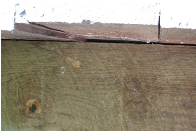
Figure 109. Deck Board Detachment
