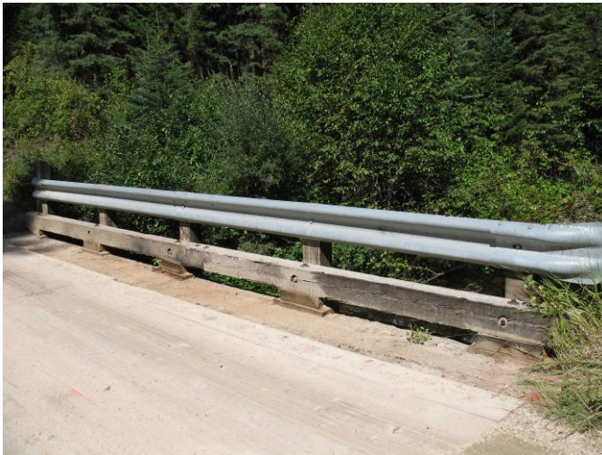
Figure 401. Burnt Fork Bridge Parapet Support
