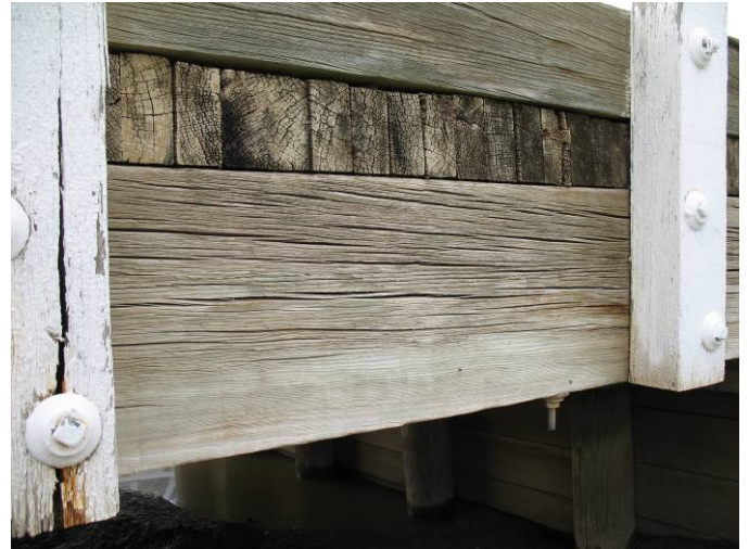
Figure 315. Checking in Exterior Girders
