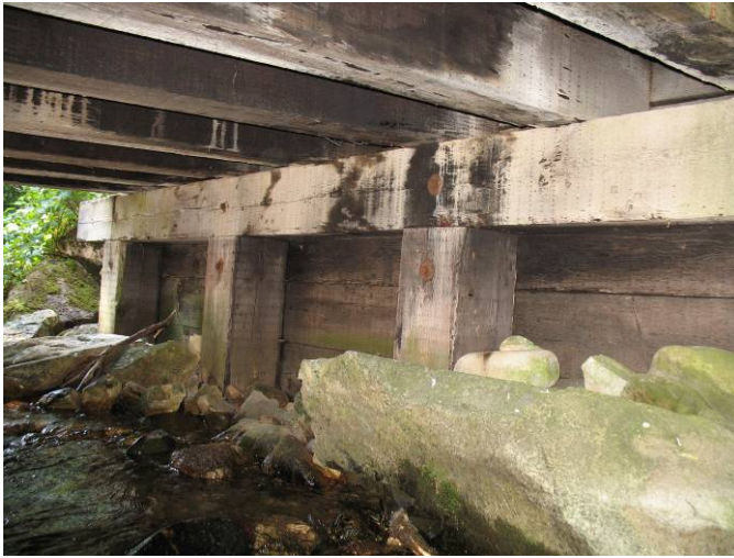
Figure 400. Bridge Substructure
