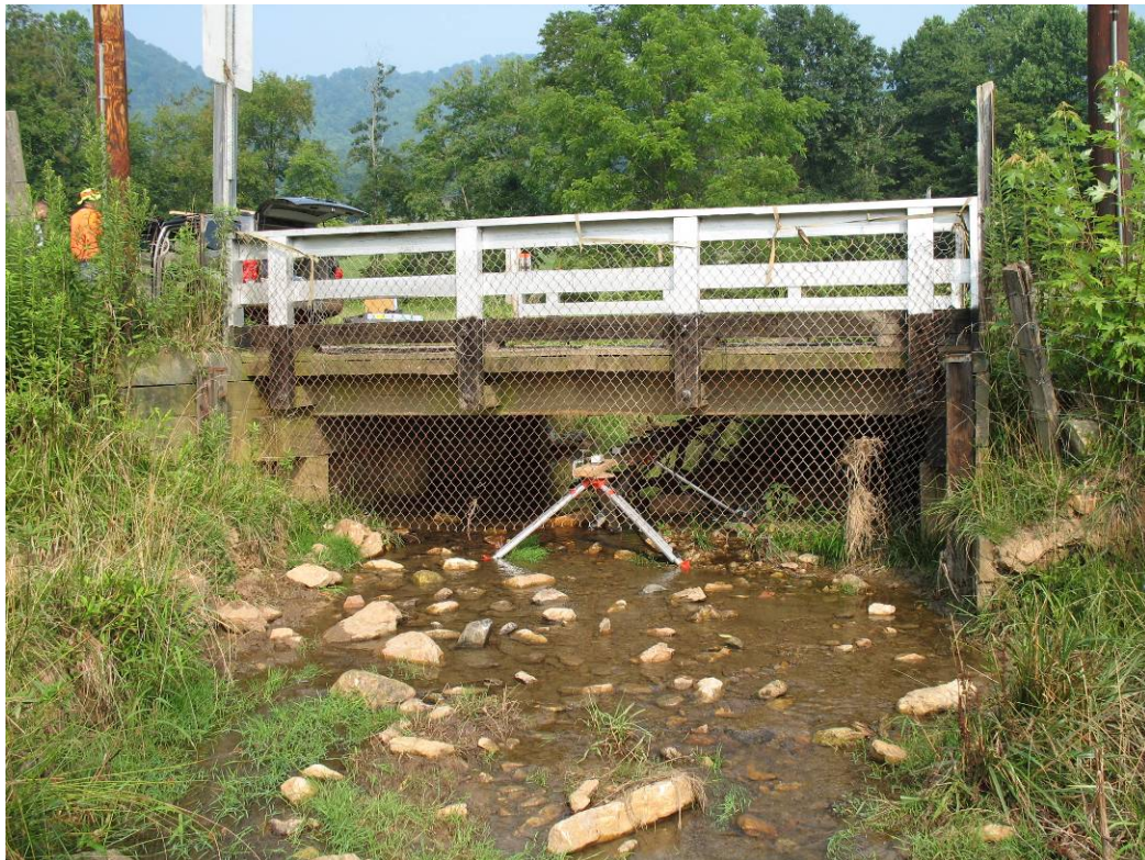
Figure 8. North Carolina Bridge used for Finite Element Modeling
