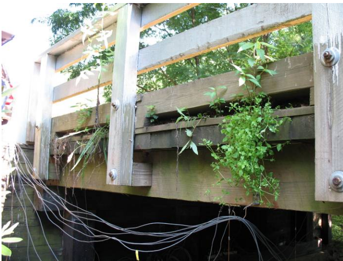
Figure 127. Dix Creek Parapet
