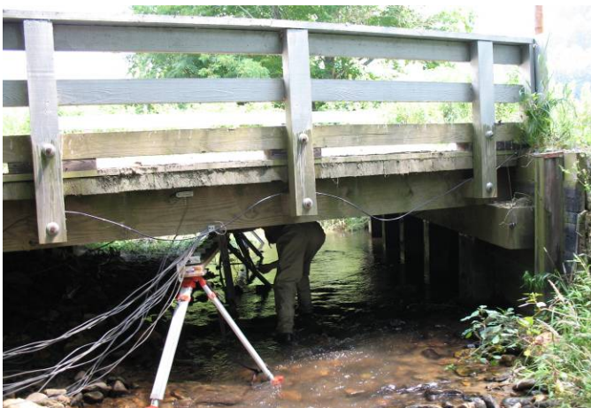
Figure 157. Bald Creek Bridge Parapet
