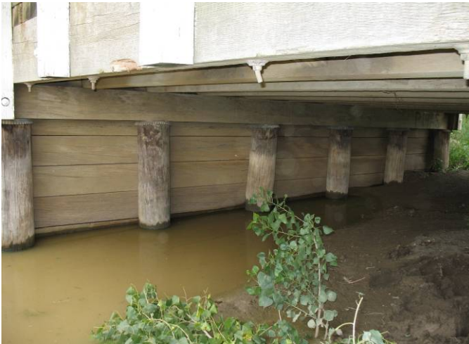
Figure 303. Bridge Substructure
