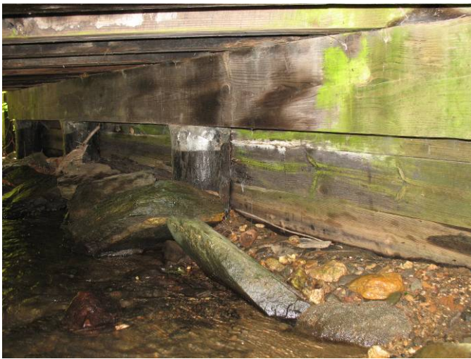
Figure 185. Substructure Sill and Posts
