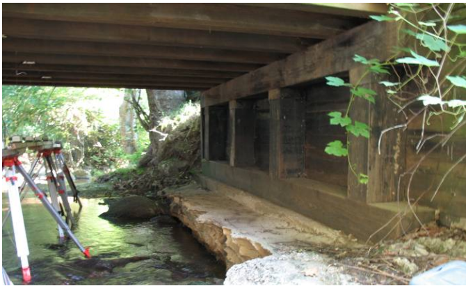
Figure 126. Dix Creek Bridge Substructure
