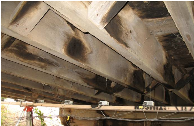
Figure 258. General Superstructure Condition
