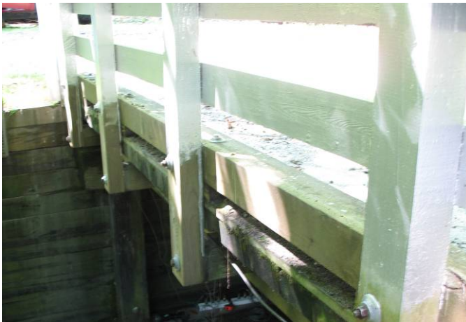
Figure 2. Chestnut Cove Creek Parapet Support
