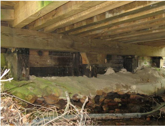
Figure 217. McDowell County Bridge Substructure
