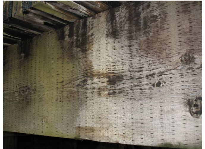
Figure 413. Checking in Exterior Girders
