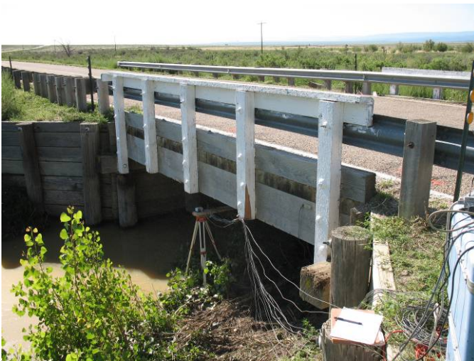
Figure 304. Colorado Bridge Parapet Support
