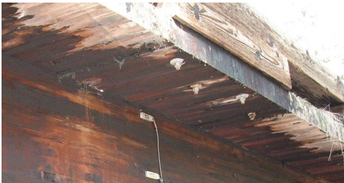
Figure 440. Washing of Creosote at Panels Ends
