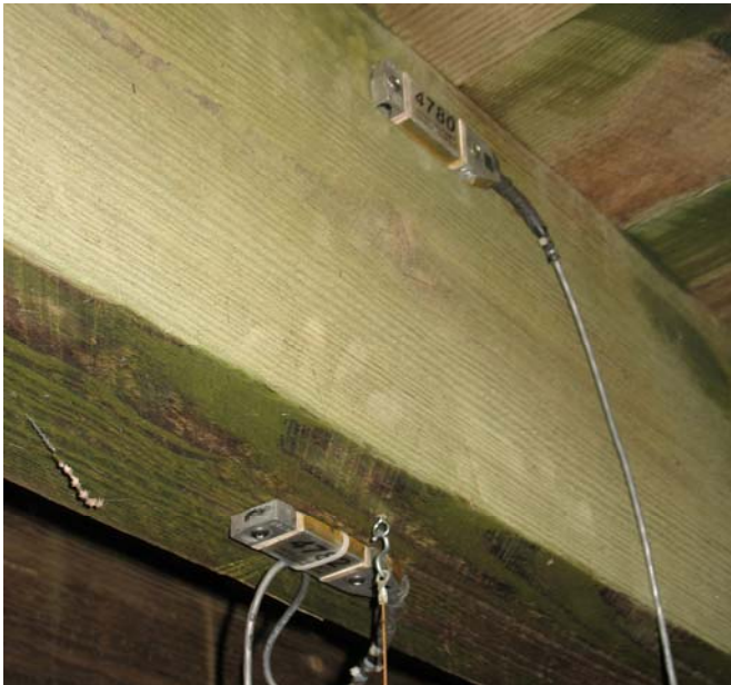
Figure 101. Outside Girder Strain Transducer Setup
