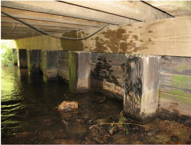
Figure 156. Bald Creek Bridge Substructure
