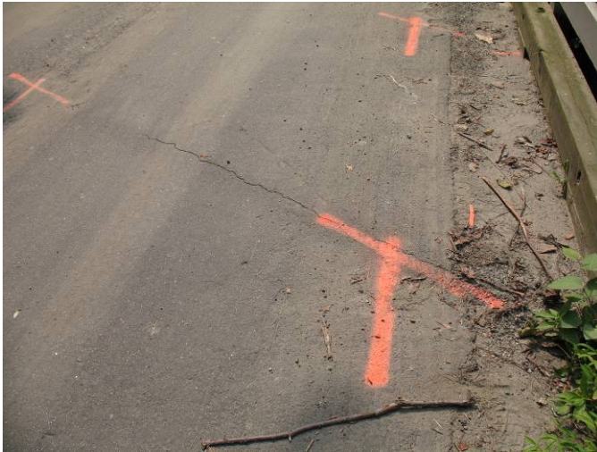
Figure 43. Transition Between Roadway and Bridge
