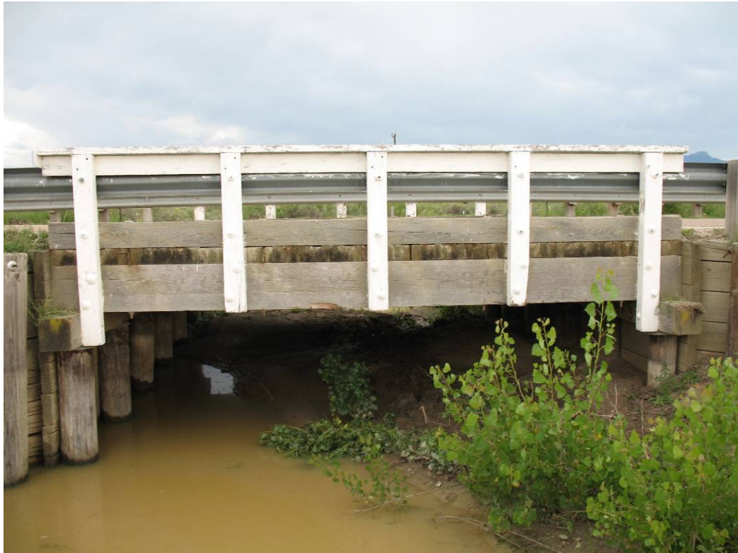
Figure 18. Colorado Bridge used for Finite Element Modeling
