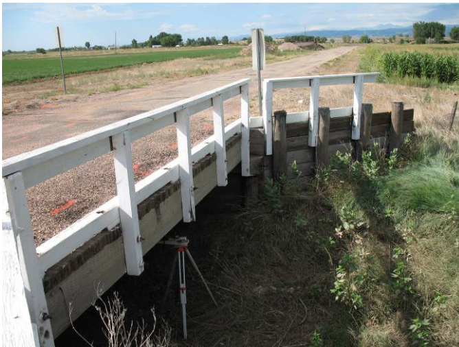
Figure 247. Larimer County Bridge Parapet Support
