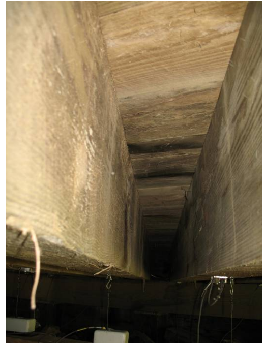
Figure 168. Typical Superstructure Condition
