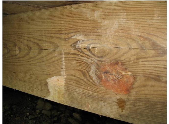
Figure 110. Checking at Girder Centerline
