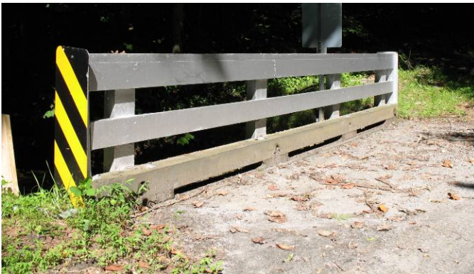
Figure 3. Chestnut Cove Creek Parapet
