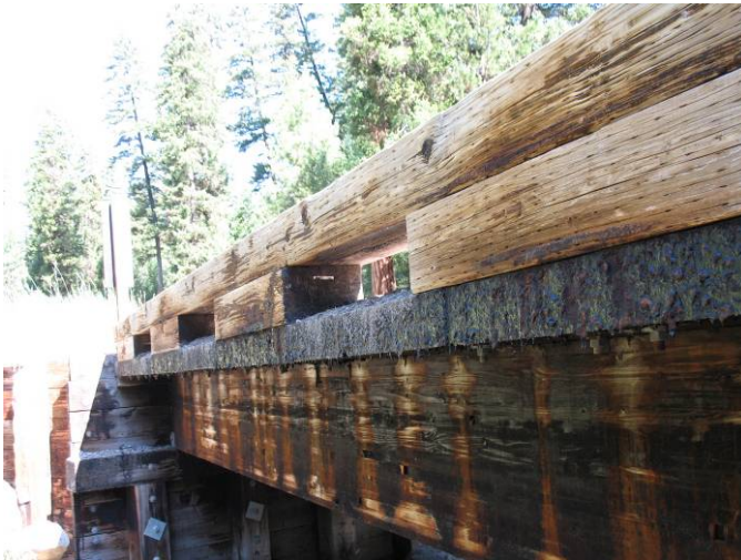
Figure 429. Trapper Creek Bridge Parapet Support
